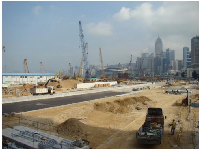
Figure 4.62: Central Reclamation Phase III
