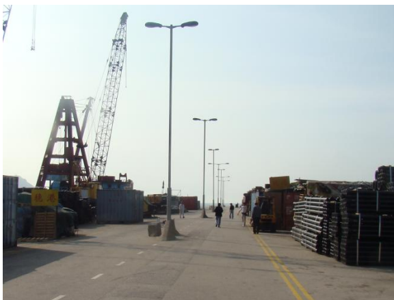
Figure 4.50: Northern Pier in Kennedy Town
