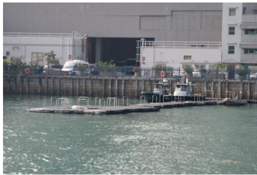
Figure 4.71: Island East Marine Police Pier
