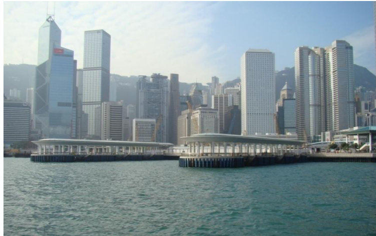
Figure 4.60: Central Piers No. 9 and 10
