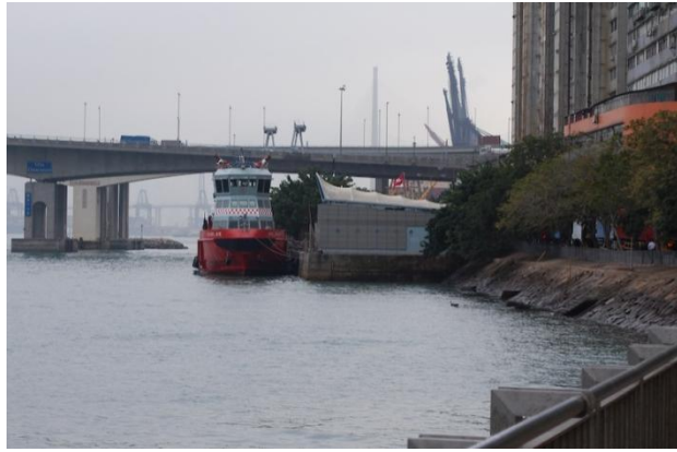
Figure 4.6: Tsing Yi Fireboat Fire Station
