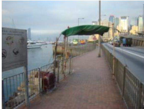
Figure 4.68: Makeshift Covered Waiting Area Next to Landing Step in Wan Chai East
