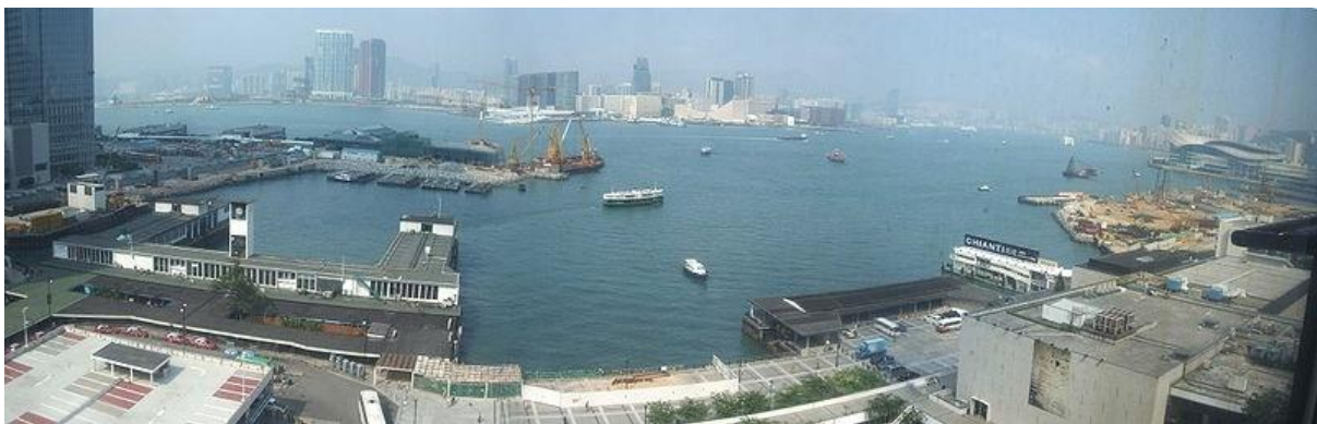
Figure 4.61: Central's Waterfront Before Central Reclamation Phase III
