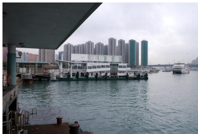
Figure 4.3: Park Island Ferry Terminal
