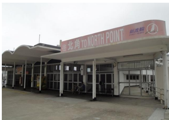
Figure 4.37: Kai Tak First Ferry Terminal
