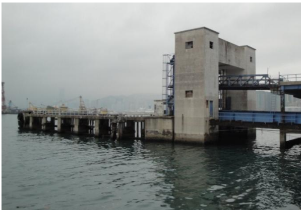
Figure 4.34: Closed-off Pier in Kai Tak
