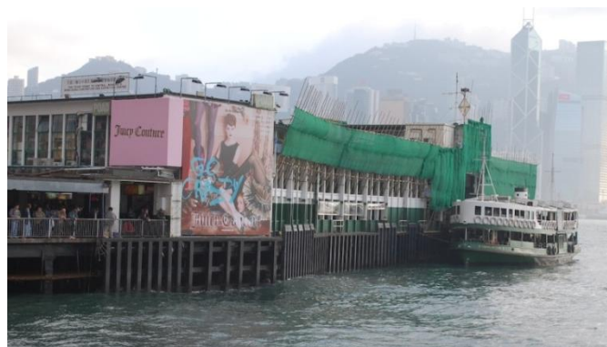
Figure 4.19: Tsim Sha Tsui East Star Ferry Terminal
