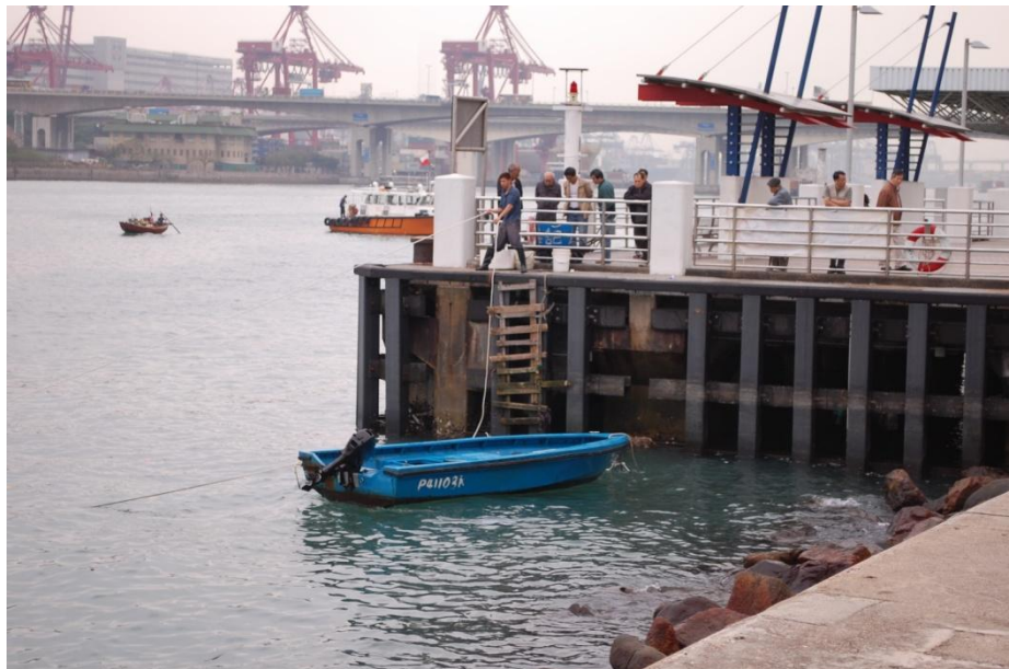
Figure 4.86: An Improvised Ladder in Tsing Yi
